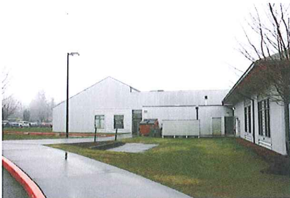
Multipurpose Building: Roof Does not Meet Current Standards for Venting
