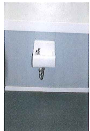
Middle School: Drinking Fountain is not ADA Accessible
