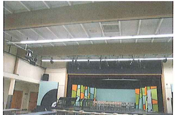
Multipurpose Building: Building is non-sprinklered
