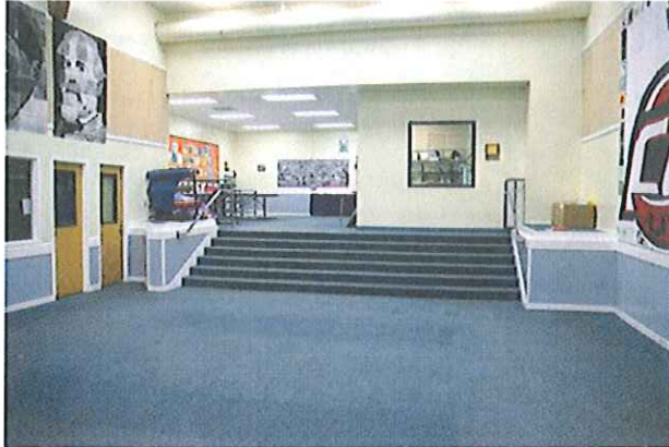
Middle School: Platform lift is Needed to Provide Accessibility to the Upper Level
