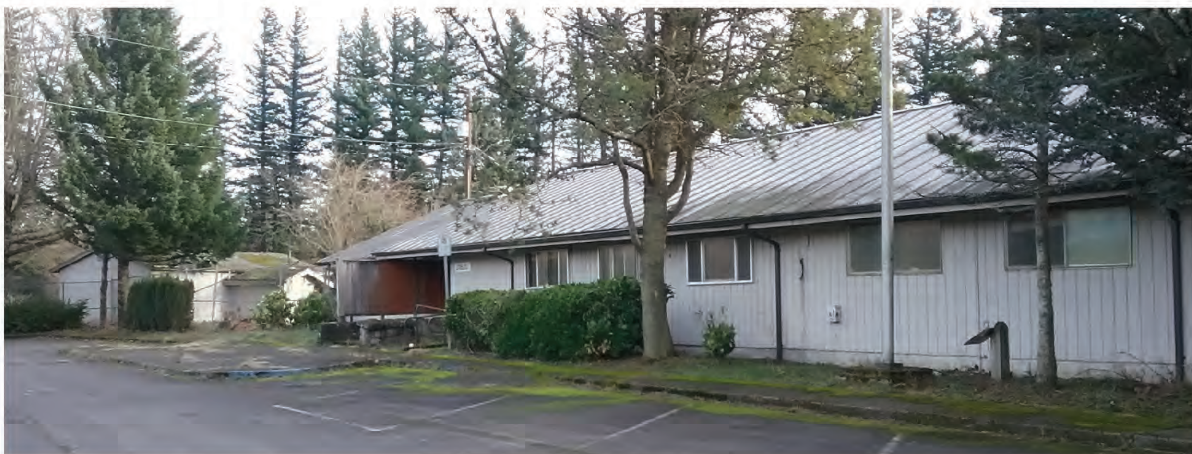
Former Reynolds Resource Center
